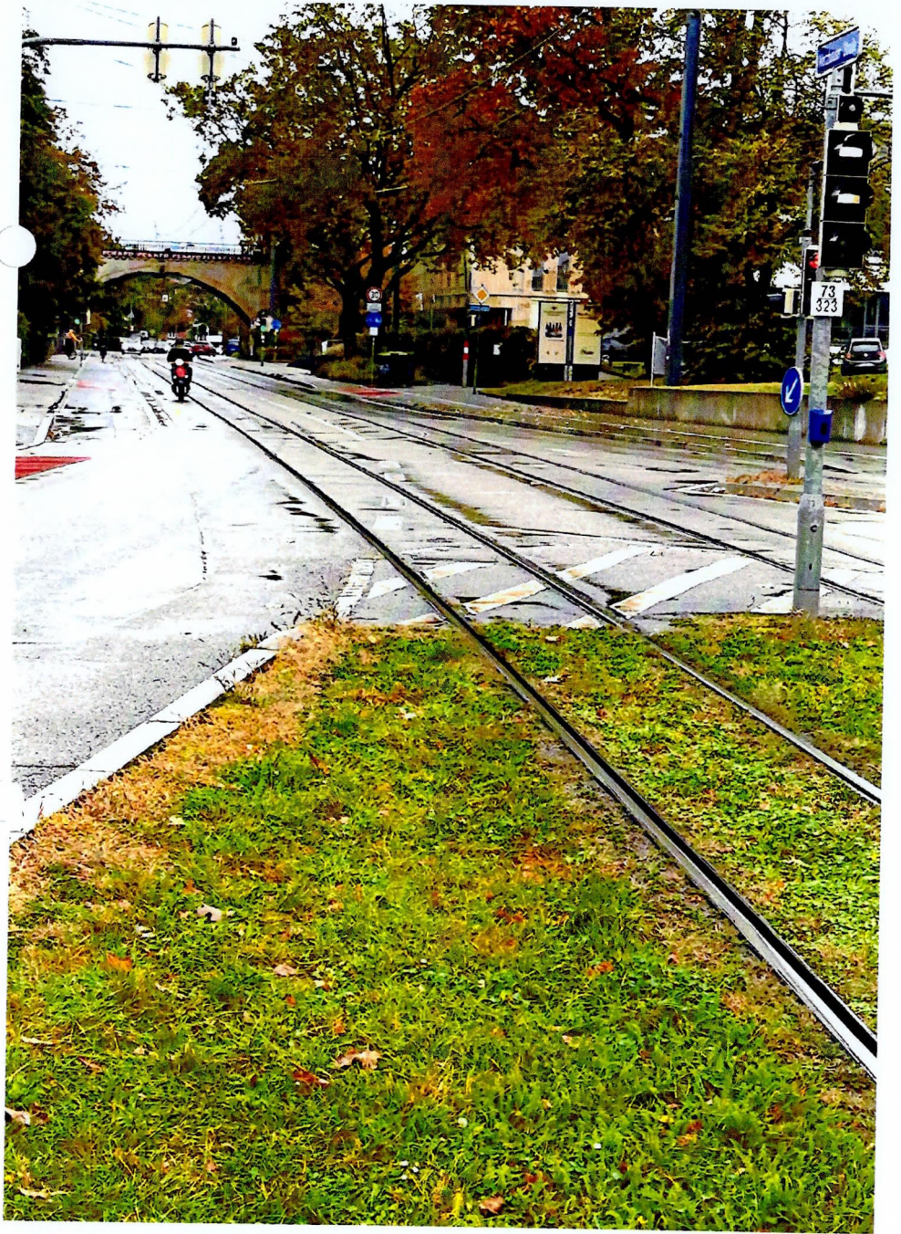
FREIBURG - CAR UNDER BRIDGE SHARES TRACK
